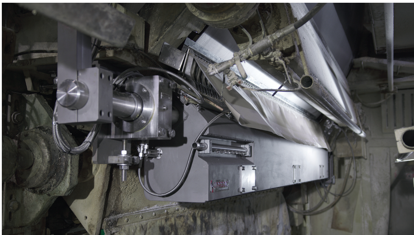
Figure 2: Overview of OraCrepe Next installation.
