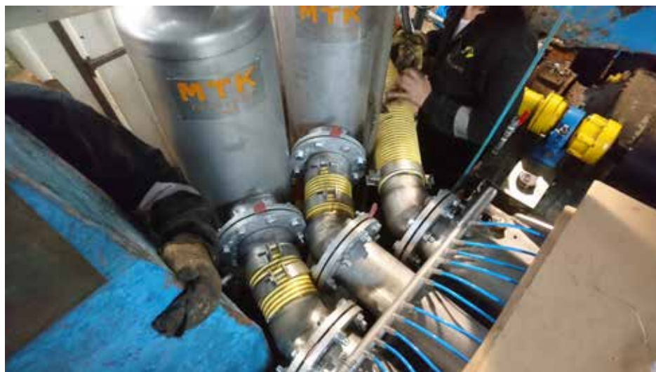
Figure 4: Trivac connection to vacuum system.
