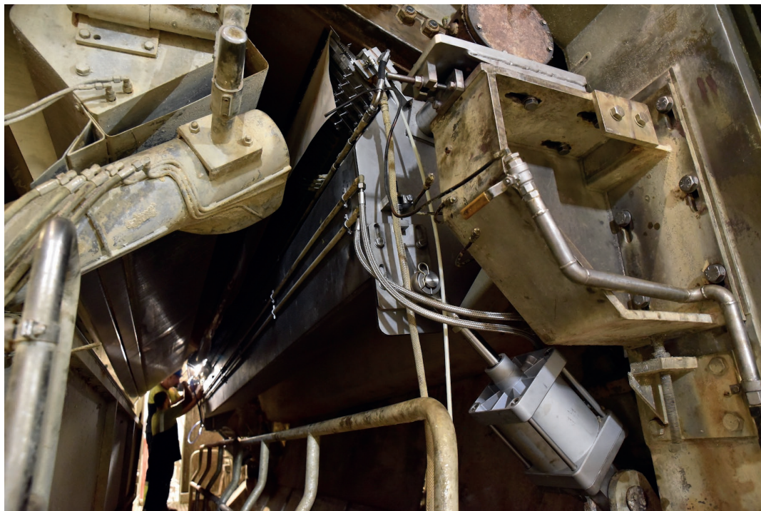
Figure 1. Creping doctor installation on Yankee.
