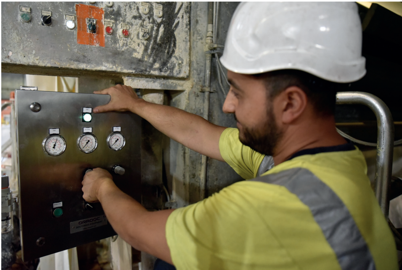
Figure 5. Essity Maintenance Leader setting pressure regulation on Oradoc control panel.
